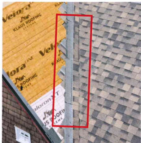
The opposite side is shingled and a leak free “California Cut” valley is created.
