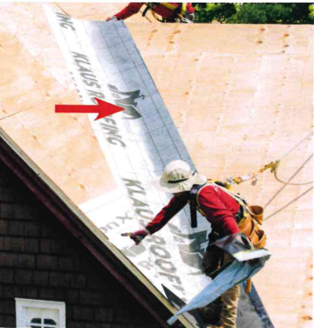
Peel-and-stick fully adhered ice and water membrane is installed 6' up from the eaves and lines the valleys.
