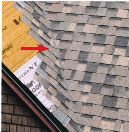
Synthetic underlayment is installed, and one side of the roof is shingled.
