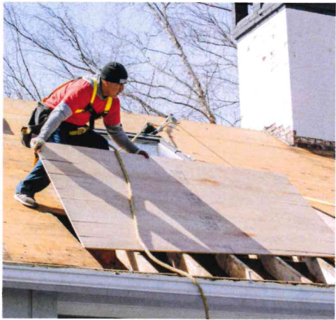
Sections of rotted roof sheathing are replaced, and existing decking is renailed with ring shank nails
